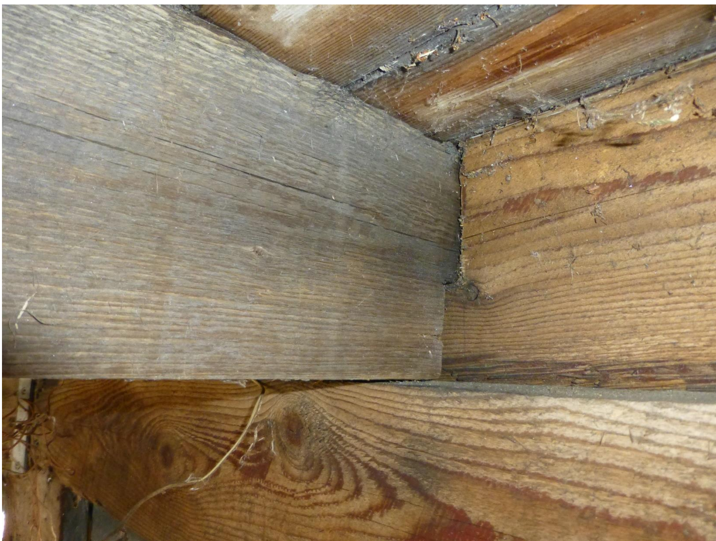
Typical joist mortise and tenoned into the 6" x 6" perimeter sill. The 2" x 6" ledger board you see under the floor joist appears to have been added later.
