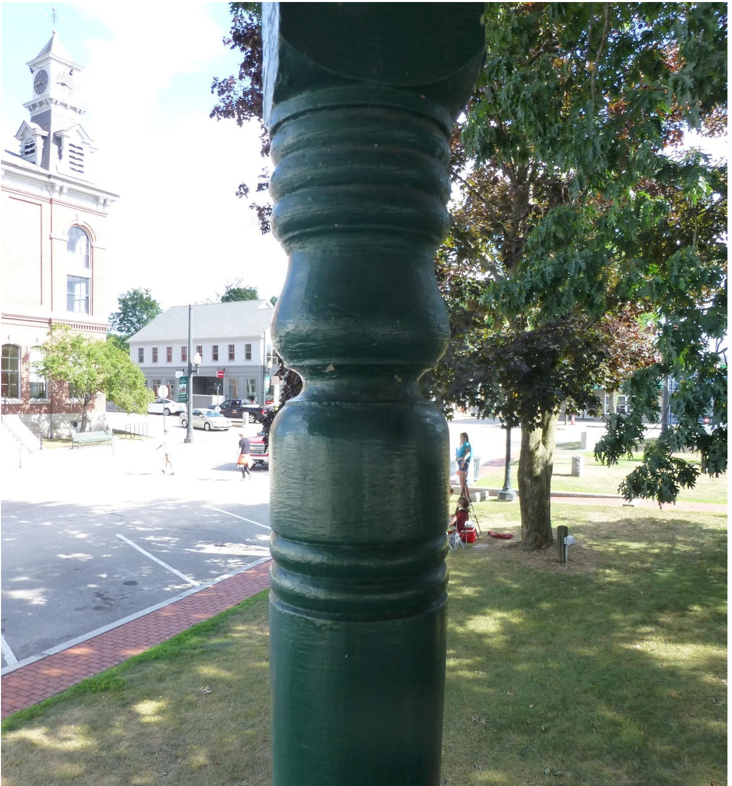
Well balanced turned details on the inverted posts, tying the upper cornice to the floor assembly.
