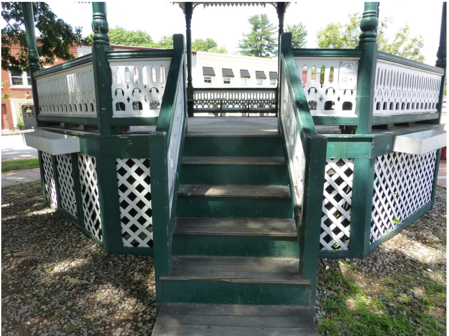
Stair entrance is in pretty good shape though will need some tread repair.
