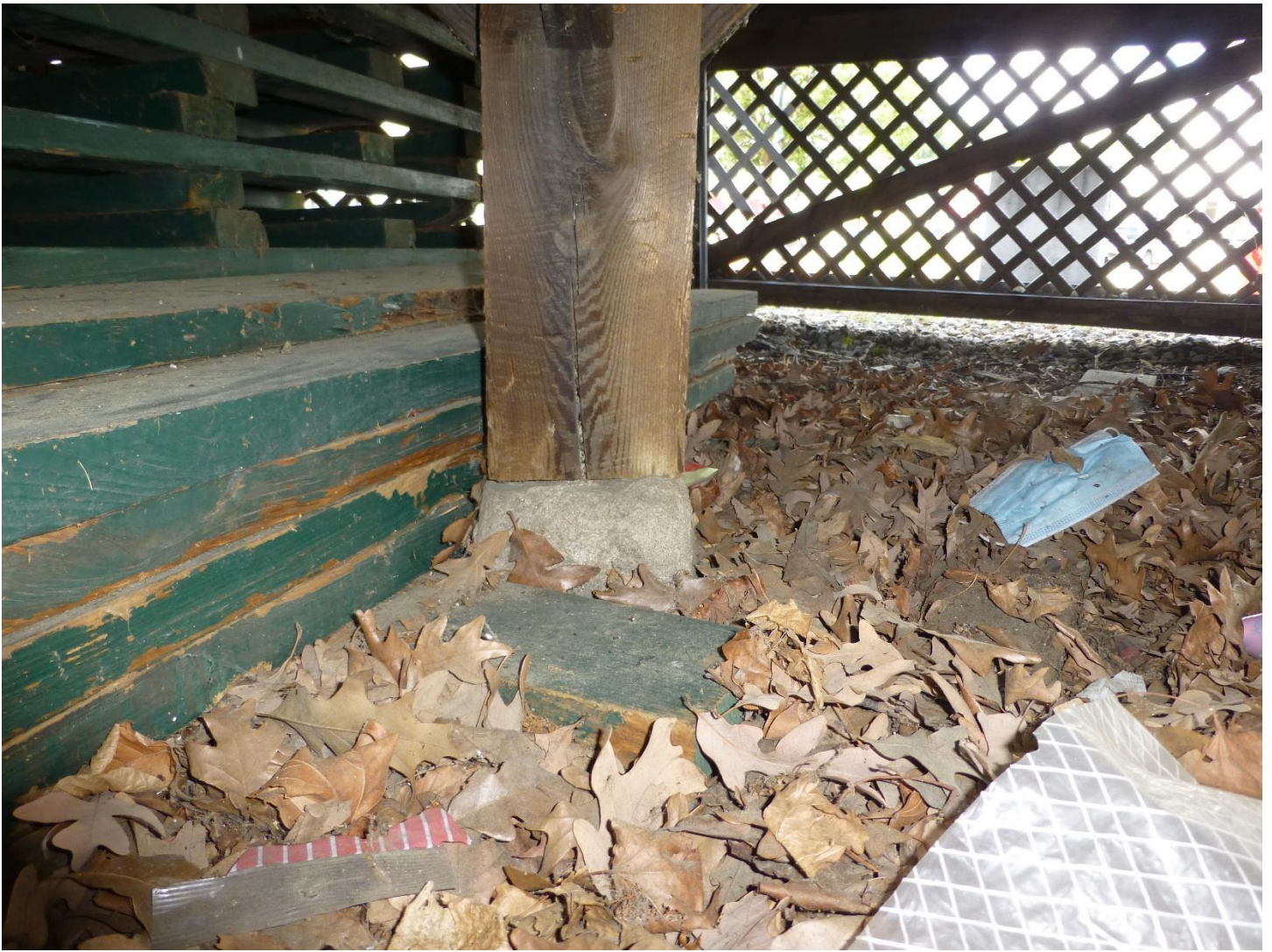
Center post and foundation stone, both appear to be in excellent condition.
