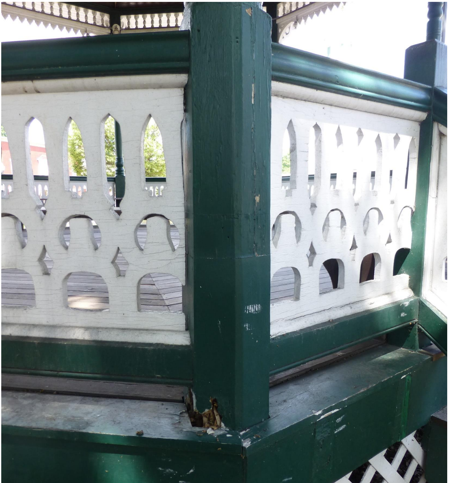
One of at least six post bottoms that need attention. It is apparent that some repairs were completed on this post the last time the bandstand was worked on.
