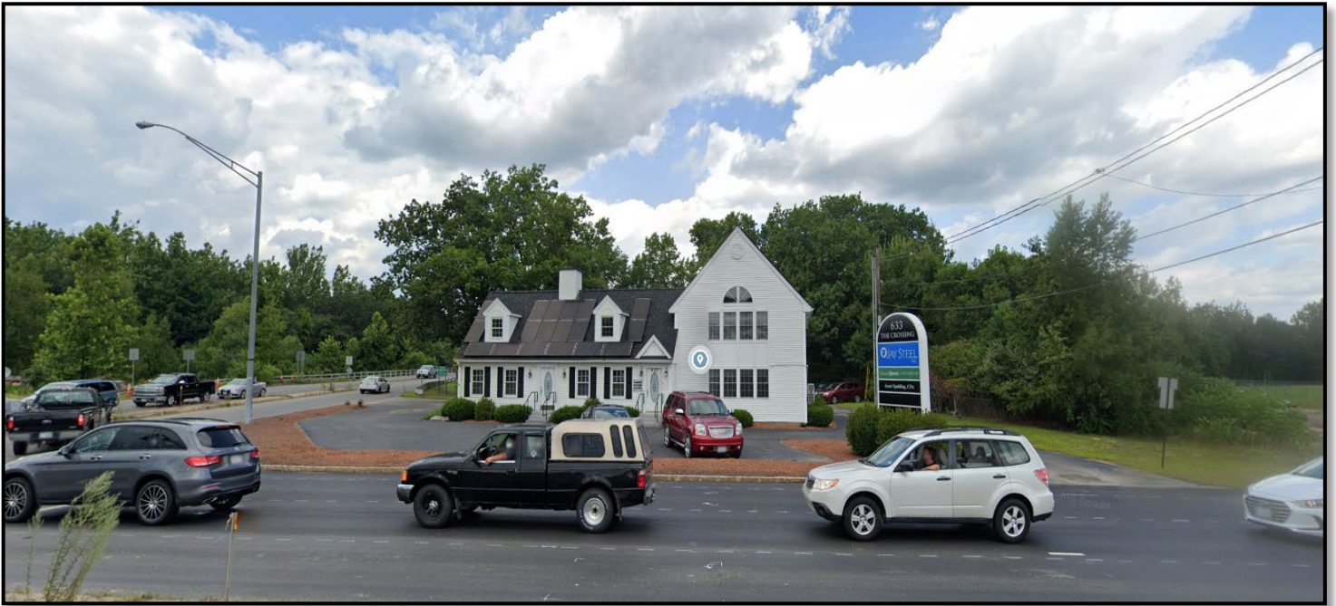
Existing Conditions (view from the south)
