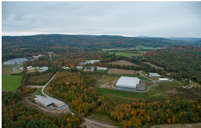
NH Industries and Davis Frame
