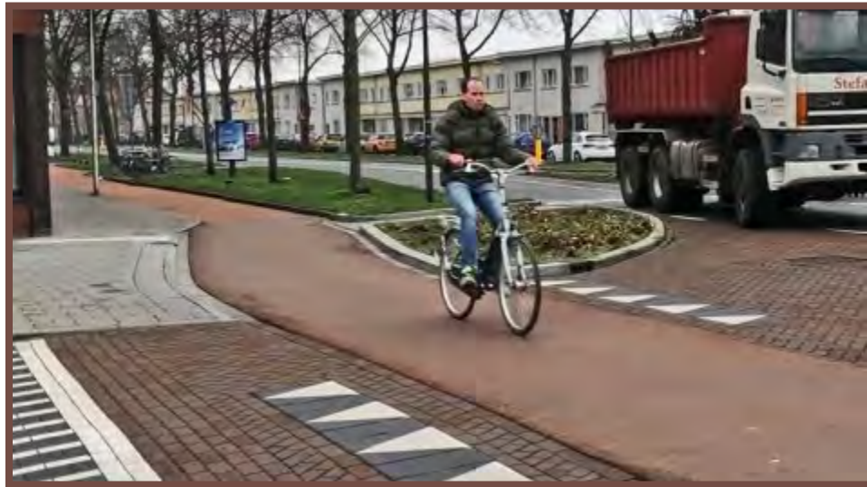
Figure 6 A sidepath/roadway intersection in which the sidepath's grade is maintained throughout (Wagenbuur 2011).
