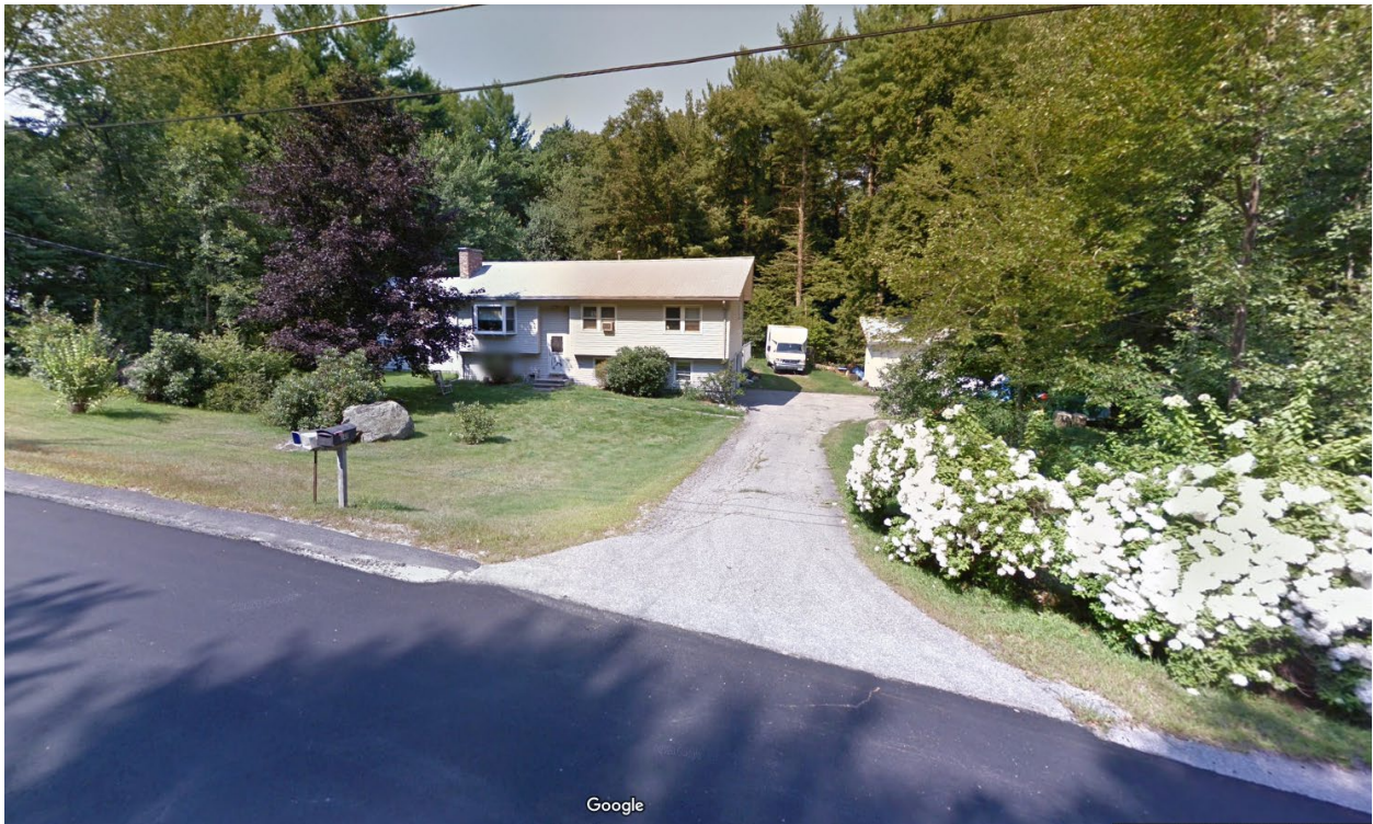
Subject Property Looking North on Comstock Drive
