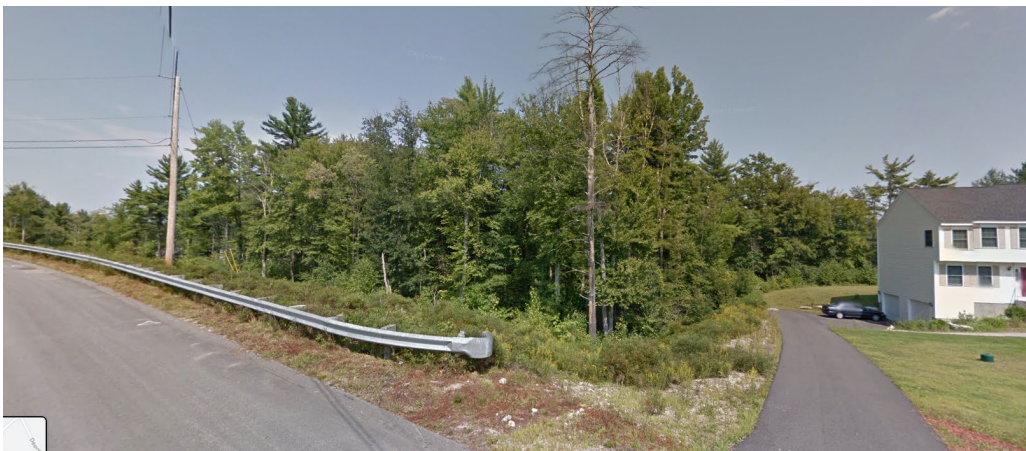
View looking Northwest on Badger Hill Drive
