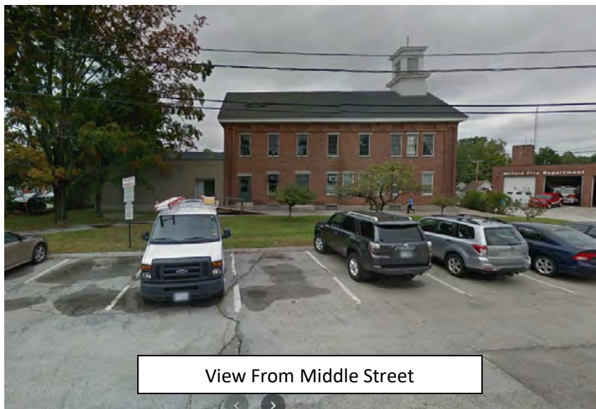
View From Middle Street
