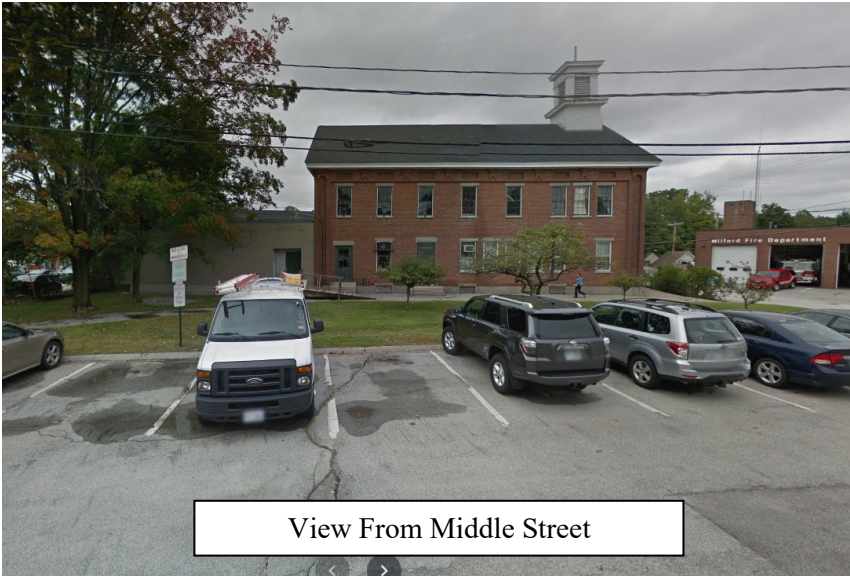
View From Middle Street
