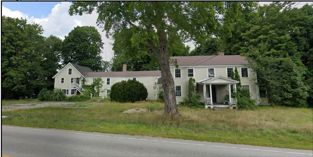
Existing (former) Conditions (has been demolished at this time)
