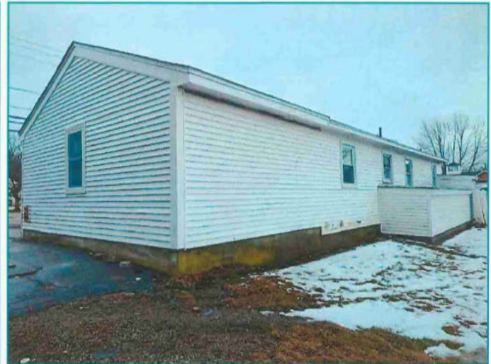
Rear of house
