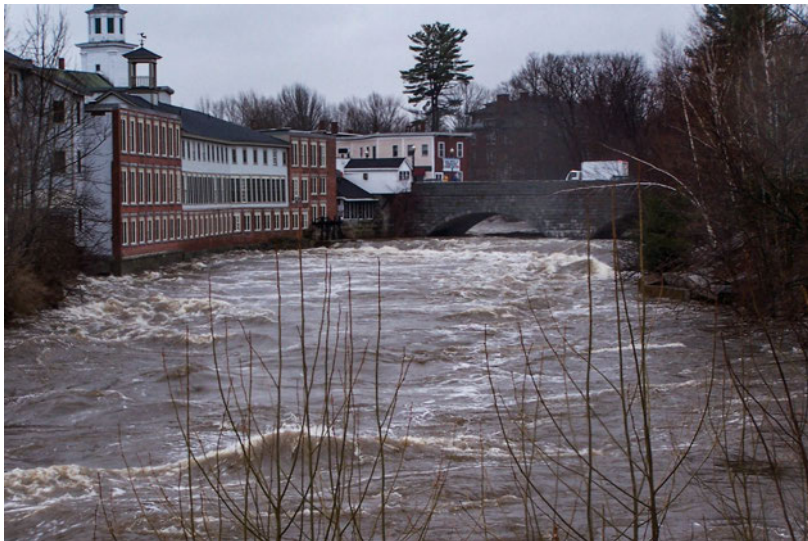
Photos: Town of Milford, NH – 2007 flood
