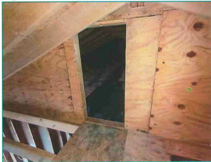
Attic access in garage.
