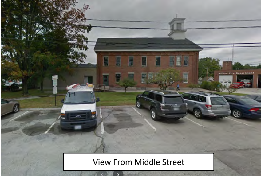
View From Middle Street
