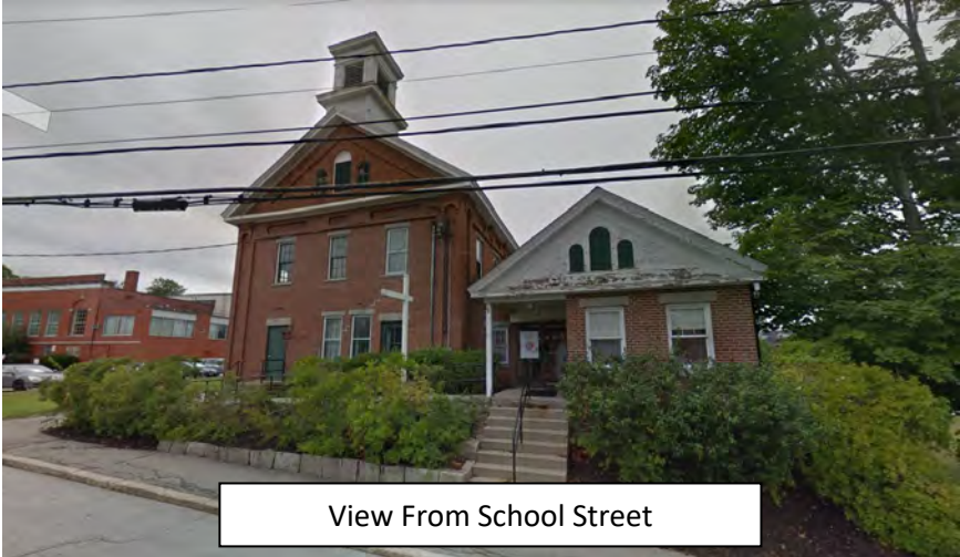
View From Middle Street
