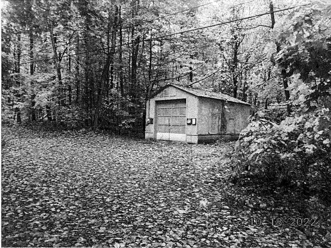
Photo 7. View north, of the garage located at the base of the access road.
