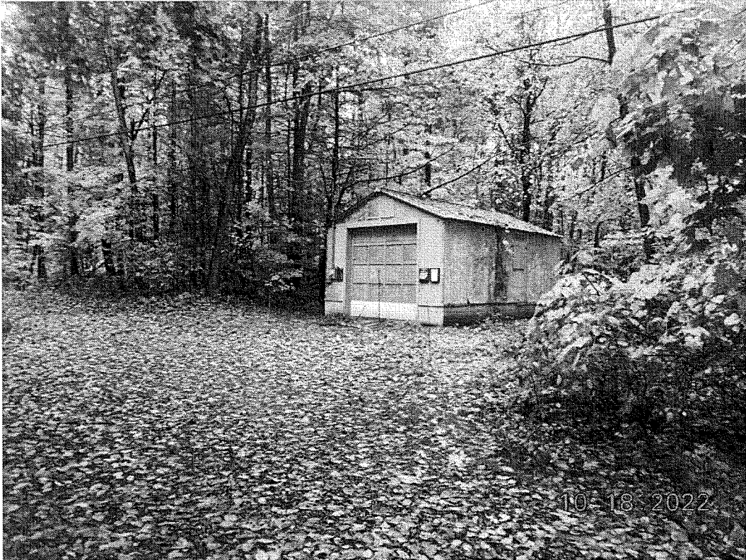
Photo 7. View north, of the garage located at the base of the access road.
