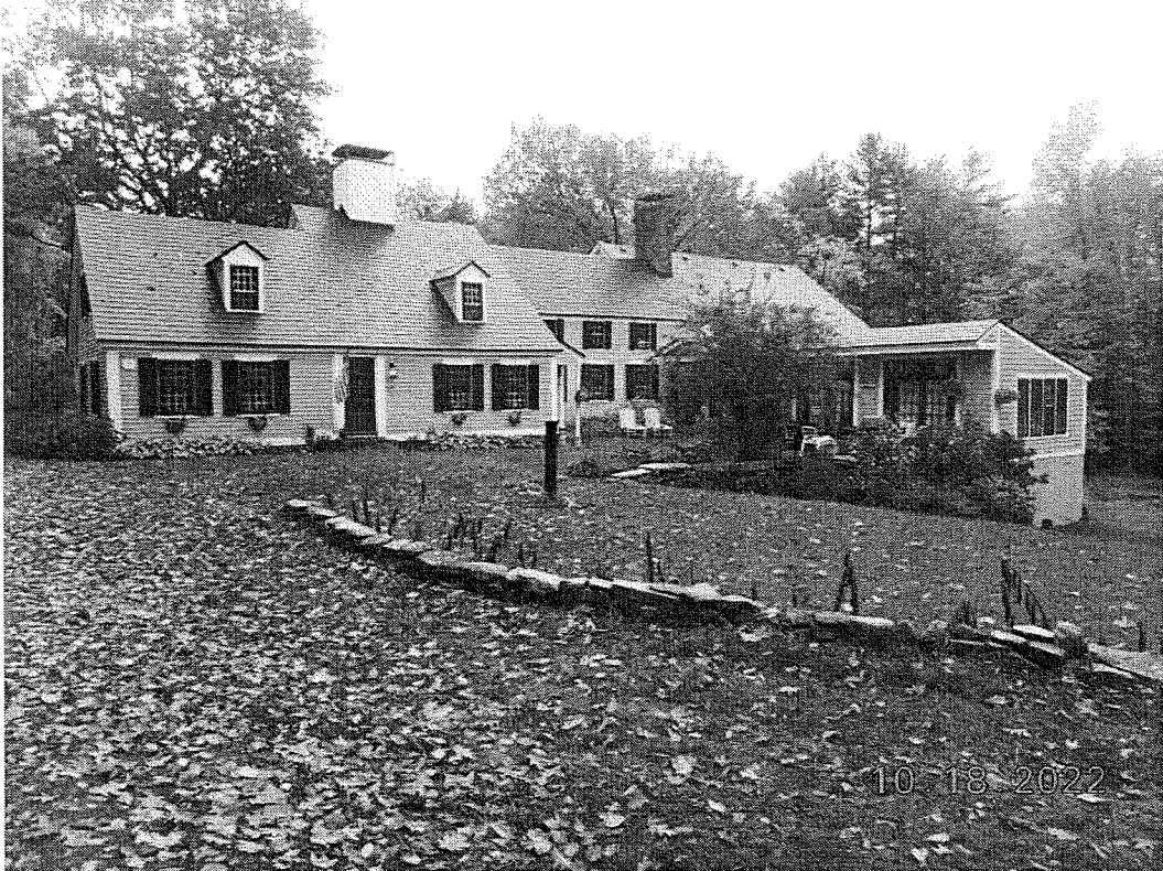
Photo 15. View northeast of 294 Ponemah Hill Road.
