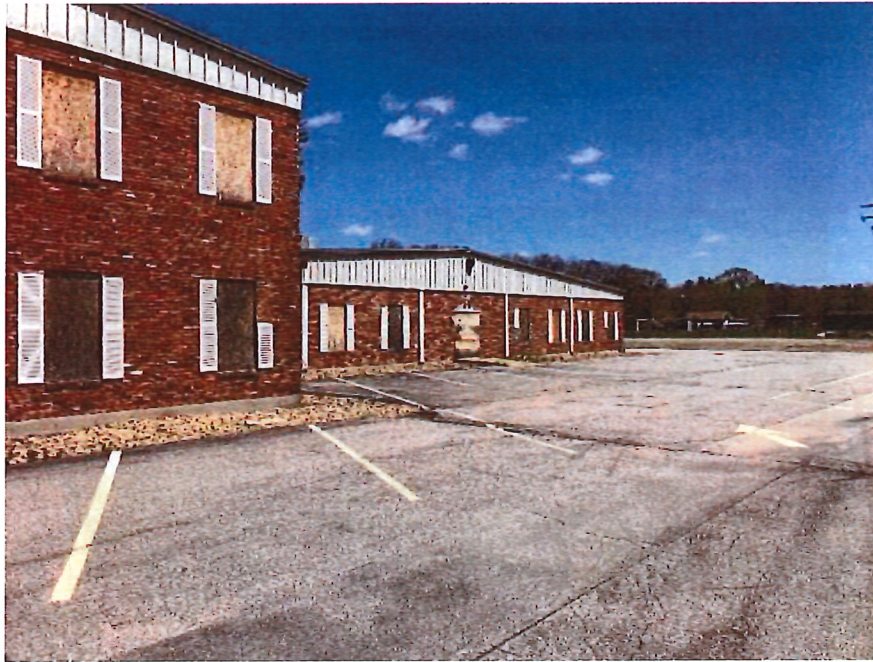
View of typical pavement condition
