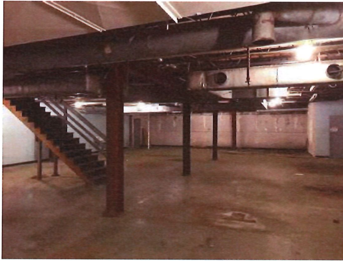
Wood stairs to second floor in middle building
