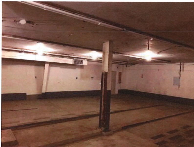
View of slab in middle building showing multiple levels
