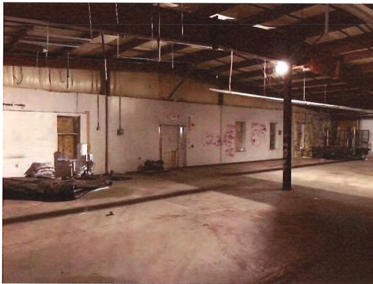
Metal building frame @ easternmost building showing columns along ridge line
