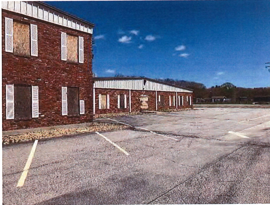
View of typical pavement condition
