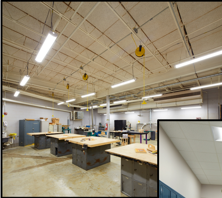
Marshwood High School Wood Shop 4Ft CLIQ Wraps
