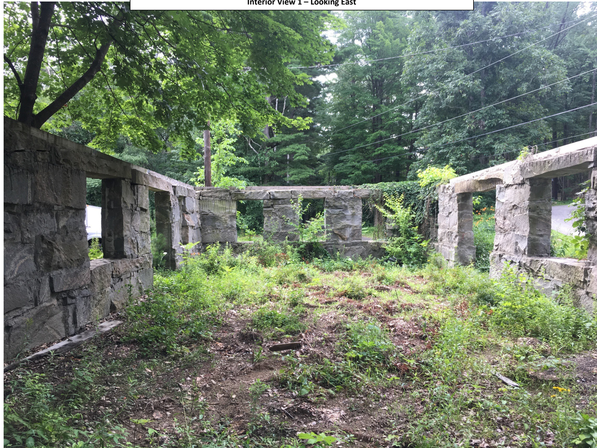
Interior View 1 – Looking East
