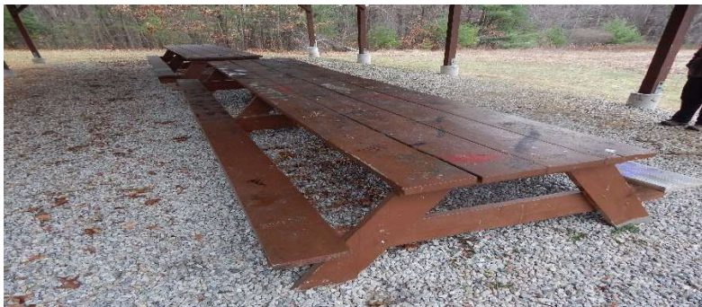
2. Graffiti and spray paint visible on picnic tables in Pavilion
