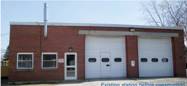
Existing station before construction
