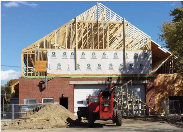
Under Construction photo taken October 2014
