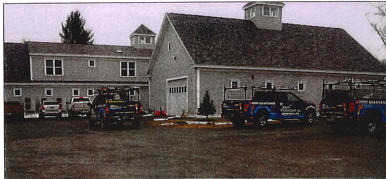
LOOKING SOUTH FROM LOCATION OF PROPOSED GARAGE ROUTE 101 IS BEYOND EXISTING BUILDING IN FOREGROUND
