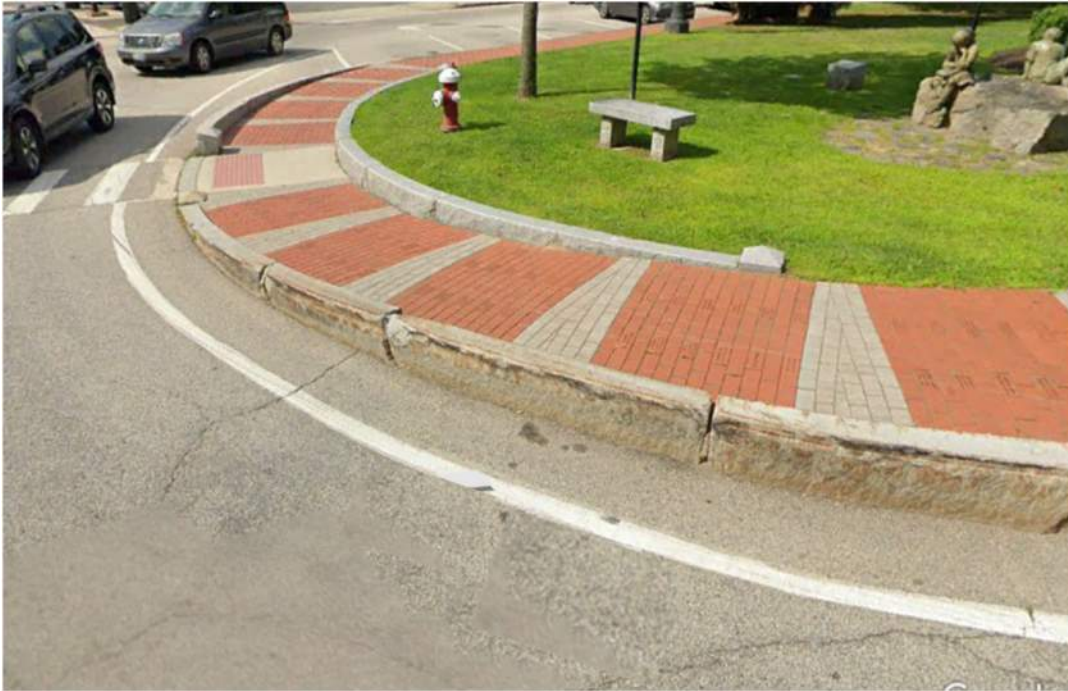
Closeup of curb damaged by truck tires at southeast corner of the Oval
