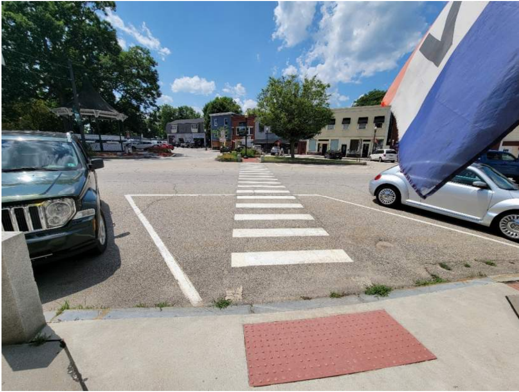
View of existing crosswalk and curb ramp looking west across northbound Mont Vernon Street
