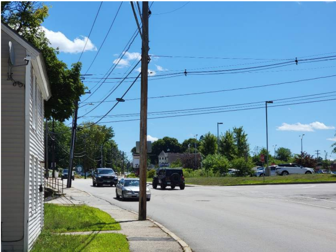
View of additional vehicles proceeding straight on Nashua Street at Clinton Street using the left turn lane
