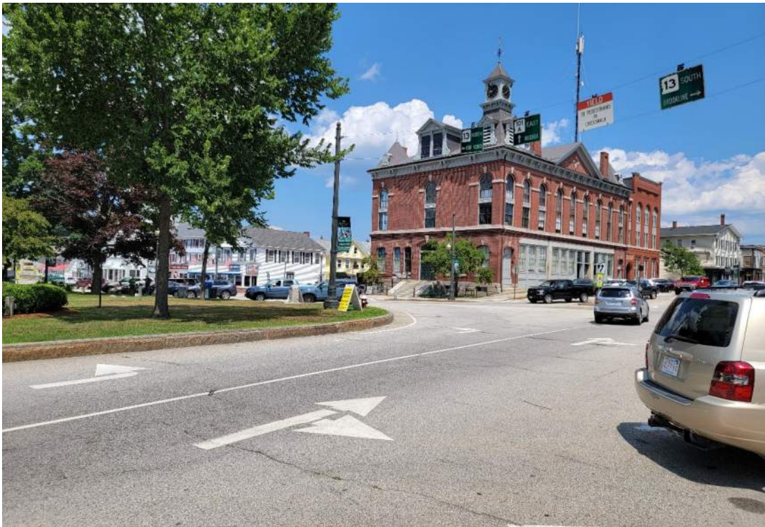
View of existing overhead signage approaching South Street and Nashua Street at the southeast corner of the Oval
