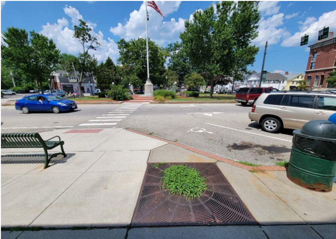
View of existing crosswalk across the south side of the Oval (Note missing tree)
