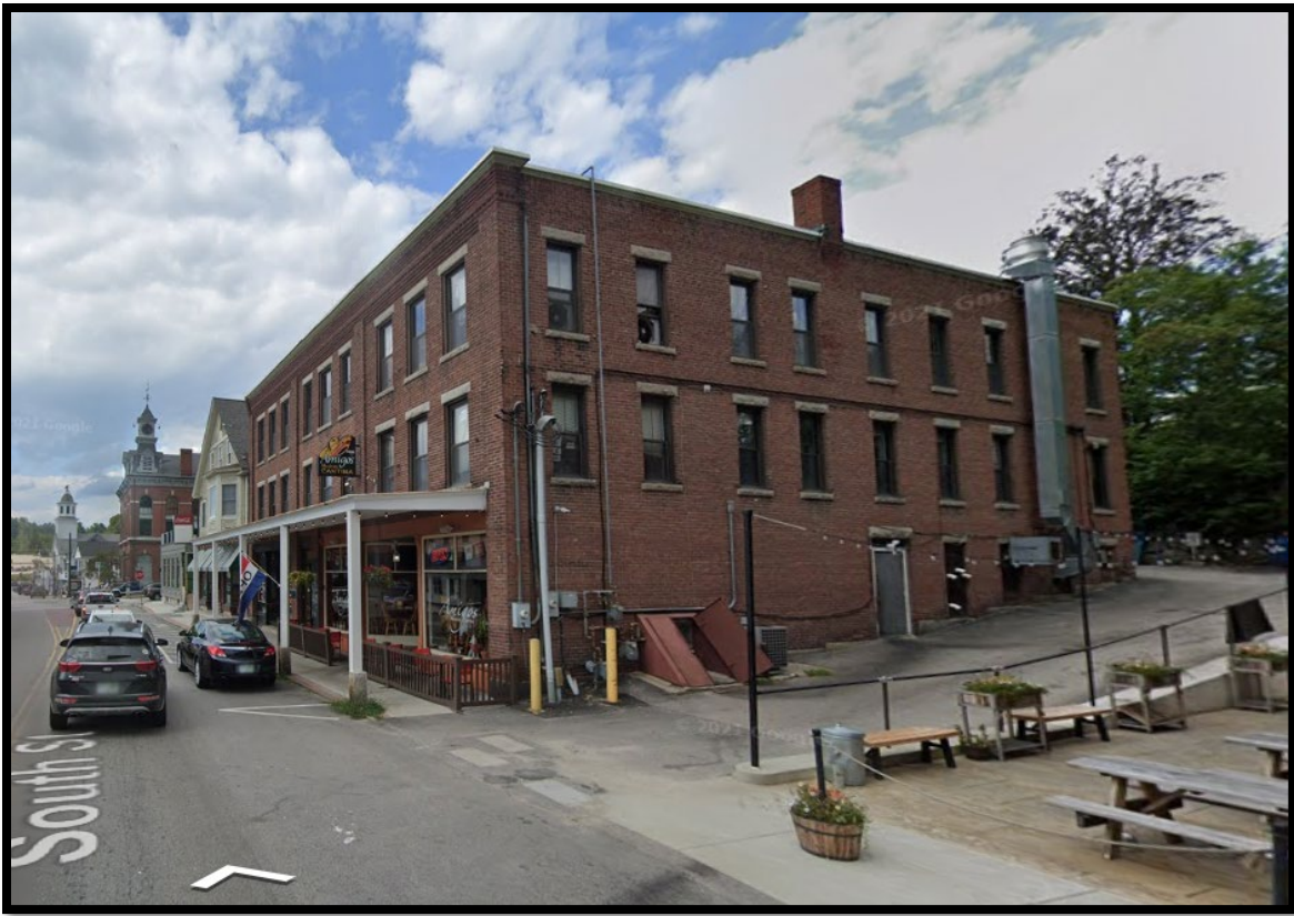
Oblique view from the south
