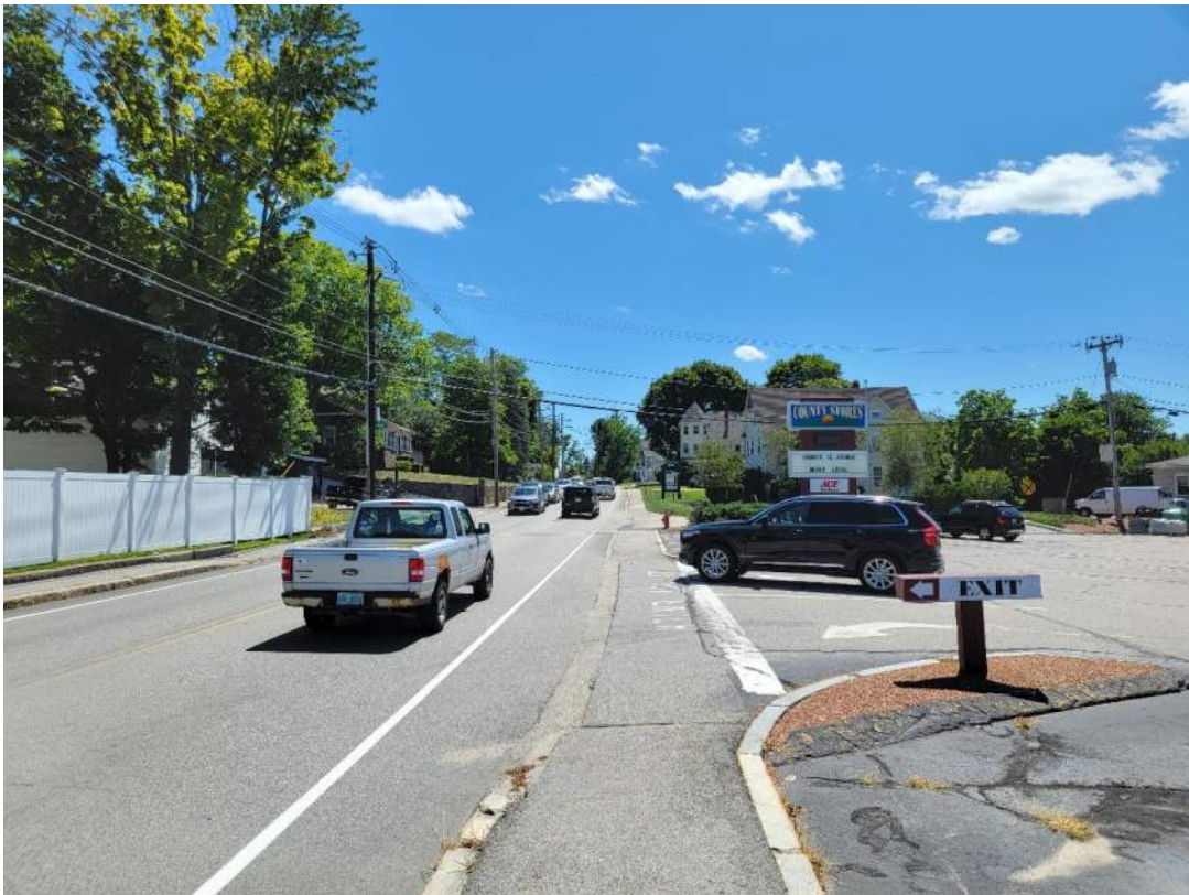
View facing southeast of the exit-only County Stores driveway from the sidewalk on the southwest side of Nashua Street
