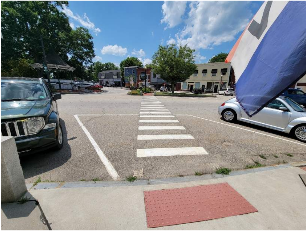
View of existing crosswalk and curb ramp looking west across northbound Mont Vernon Street
