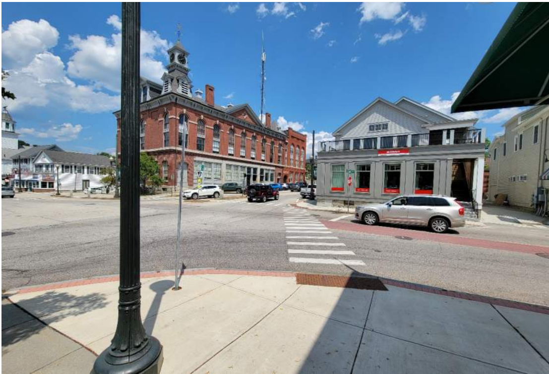
View across South Street looking toward Nashua Street, at the southeast corner of the Oval
