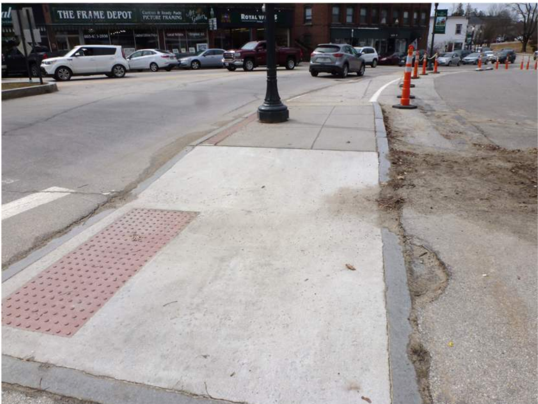
View facing southwest toward Union Street with the Riverhouse Café and the long curb cut to the Station 101 parking lot to the right.
