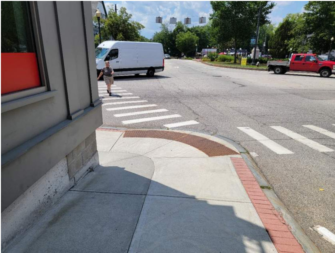
View of existing curb ramp at southeast corner of South Street and Nashua Street, looking west into the Oval
