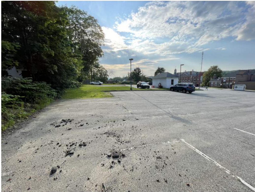
View facing west to rear portion of library site where future parking lot expansion is planned. Note that white storage building will be removed, and a new storage shed will be placed at the southwest corner of the site.
