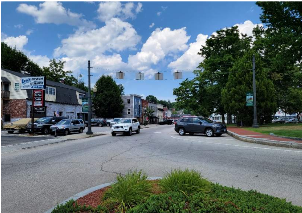
View northeast along the west side of the Oval from the Elm Street median island
