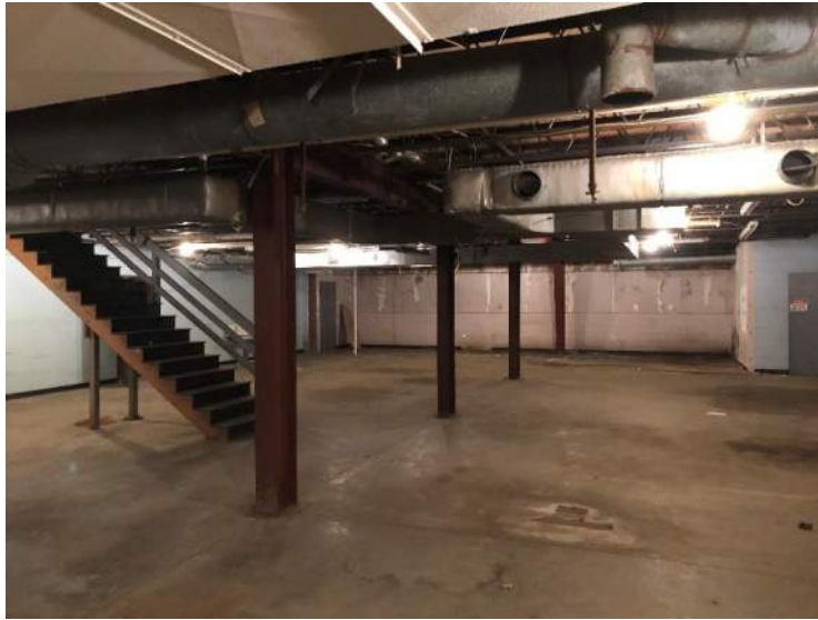
Wood stairs to second floor in middle building
