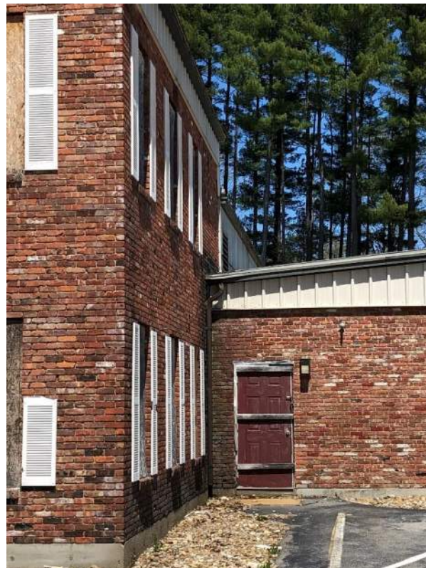
View of roof pitching into sidewall
