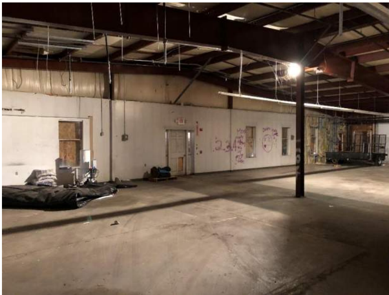
Metal building frame @ easternmost building showing columns along ridge line
