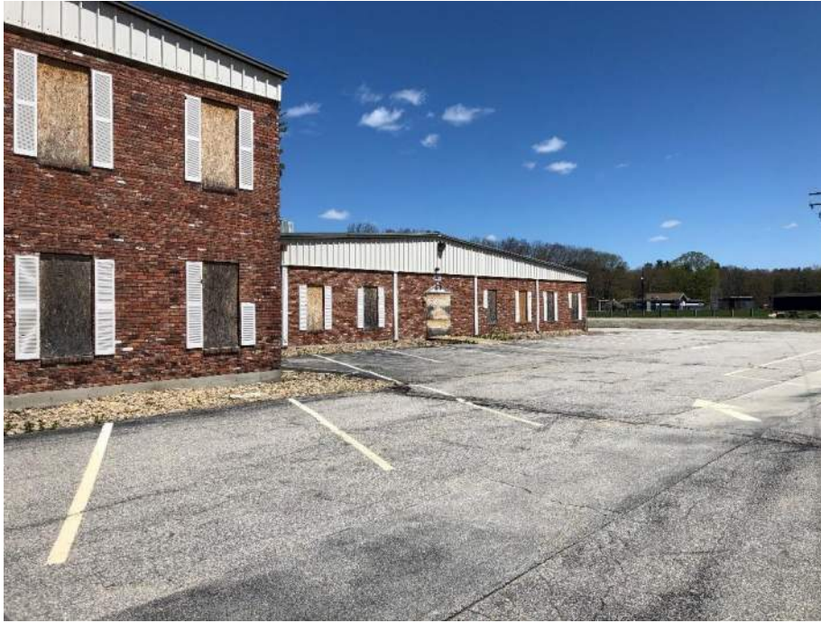
View of typical pavement condition
