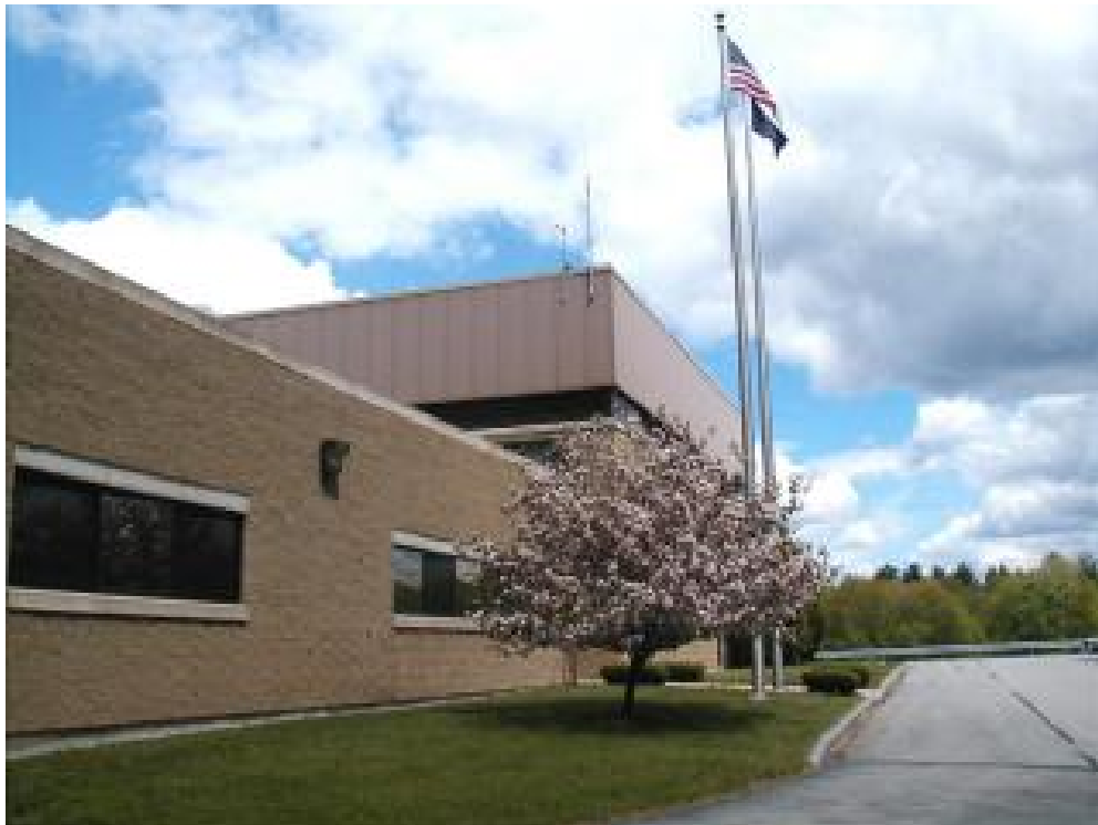
Water Utilities Building
