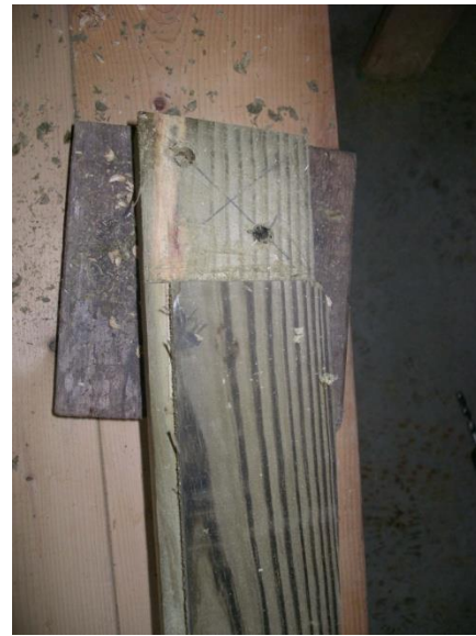
Photo 2-4: Location of holes for lag screws
