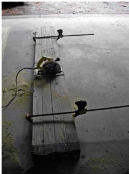
Photo 2-1: Cutting Grooves
