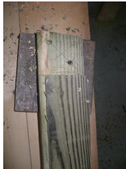
Photo 2-4: Location of holes for lag screws
