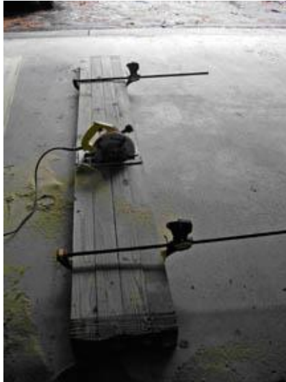
Photo 2-1: Cutting Grooves
