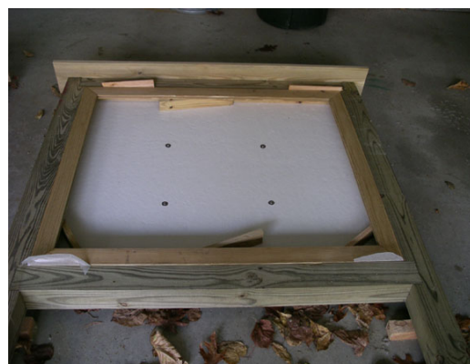
Photo 2-6: Homosote screwed in place. Window frame in position supported by spacer scraps.
