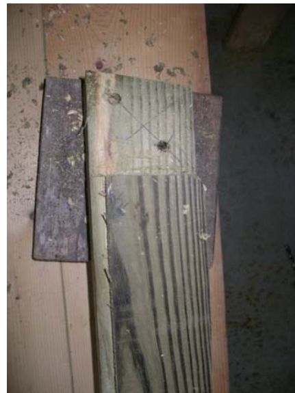
Photo 2-4: Location of holes for lag screws
